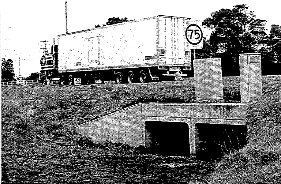
Figure 2. CULWAY WIM site
