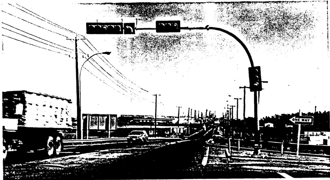
TRAFFIC CONTROL SIGNAL WITH ROTATABLE BASE
