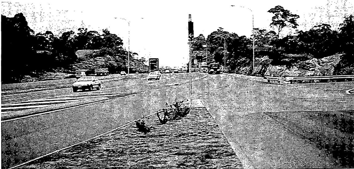
Figure 6. View of the HSEMU weigh plates and traffic lights from control room
