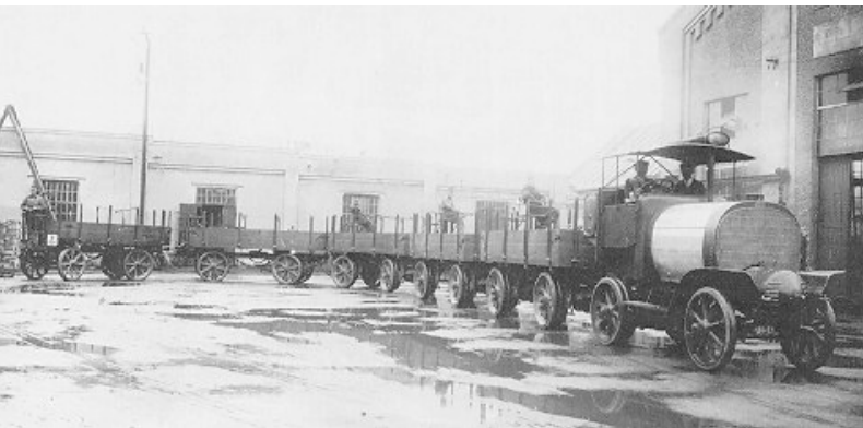
Figure 1. Five-trailer all wheel steering vehicle (1911).
