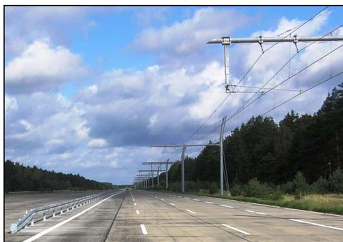
**Figure 5 – Overhead contact line, roadway and protective equipment**
