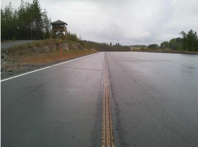
**Figure 4 - The Elways electric beam on a test site.**
